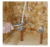
4. Disconnect and remove the hot and cold water feed lines from the water supply valves.
