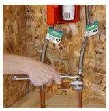
**NOTE:** The Hot Water Lobster has two 12" flexible cold water lines and two 12" flexible hot water lines preassembled. If necessary longer water lines or adaptors may be purchased at your local hardware or plumbing supply store.
