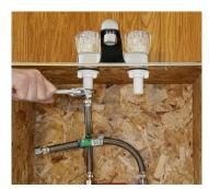
6. Connect and tighten the ½" brass pipe thread fittings snugly to the faucet (hot to hot & cold to cold). **NOTE**: Do not over tighten. The brass fittings have rubber seals (do not use pipe compound or Teflon tape).
