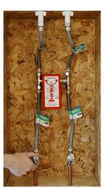
8. FIRST: Turn on the hot water supply valve only, then turn on the cold water side of the faucet only. Wait until water flows from the faucet (turn off after about 6-seconds). NOTE: If the water in the pipe is hot, the water may have to cool down before water will flow through the faucet. SECOND: Turn on the cold water supply valve to the faucet. THIRD: Installation is complete and the faucet may be used as normal.
